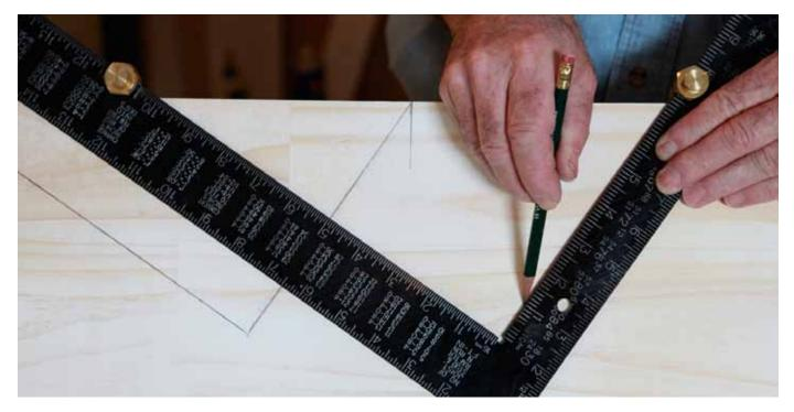
To make it easier to install the stringers, Mike Sloggatt likes to cut the stringers so the tops register off the bottom of the deck joists. In the set we use for our clinics, the joists are only 2×4s (it's just a set!),
