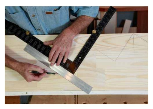
Using the story pole is the easiest way to avoid a bottom riser that's too tall and ensure that the stringer sits right on the rough concrete pad. With that detail completed, the template can only be used for rough-to-rough layout.
