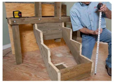
The decking and treads are 1 in. And the stone or brick added later will be 2-1/2 in. thick.
