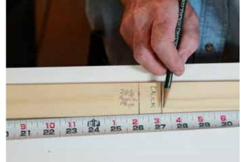
Divide that measurement by the total number of risers. Because the maximum rise allowed by IRC code is 73/4 in., in this example we use 4 risers.
