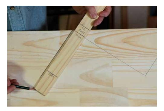
Then extend that line across and beneath the first tread—that's the line of the concrete pad.
